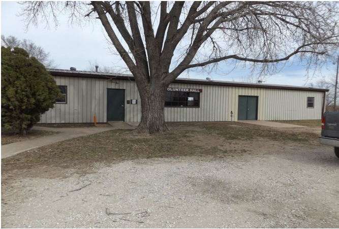
Front View—Single and Double door entrances. Views of lake. Boat ramp, swim beach, and playground near by.
